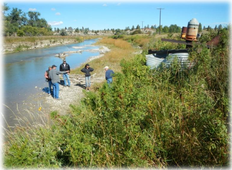
Figure 5. Perched pump site upstream of breached diversion dam.
