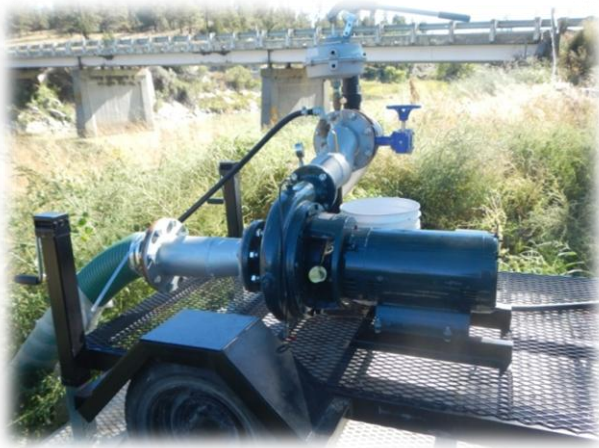
Figure 2. Pump site below highway bridge.
