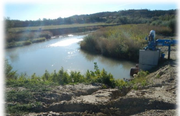
Figure 1. Newly reconstructed pump site downstream of Roundup.
